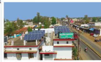
Solarization of a health centre, Chhattisgarh
